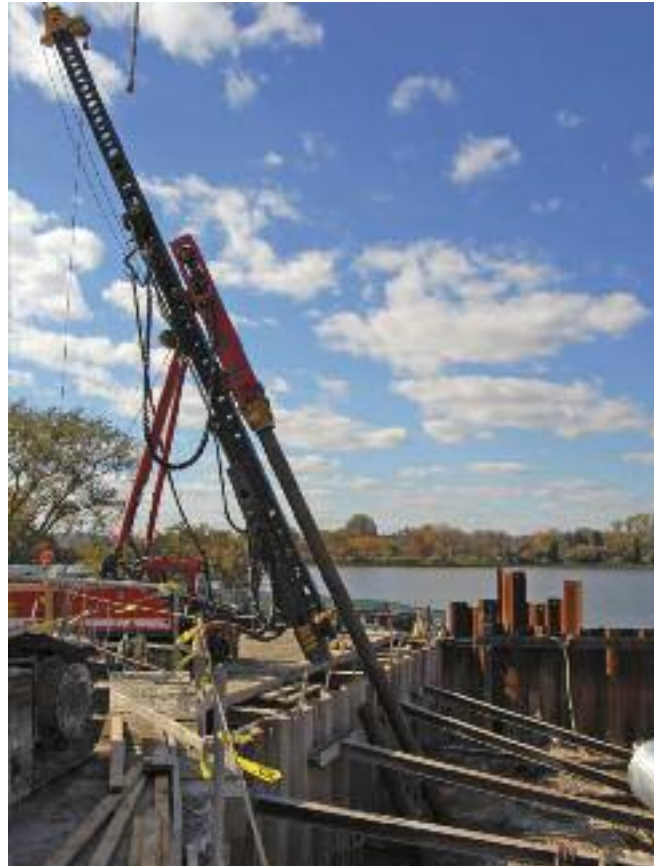
Pile driving rig reaches over to install battered pipe piles.
