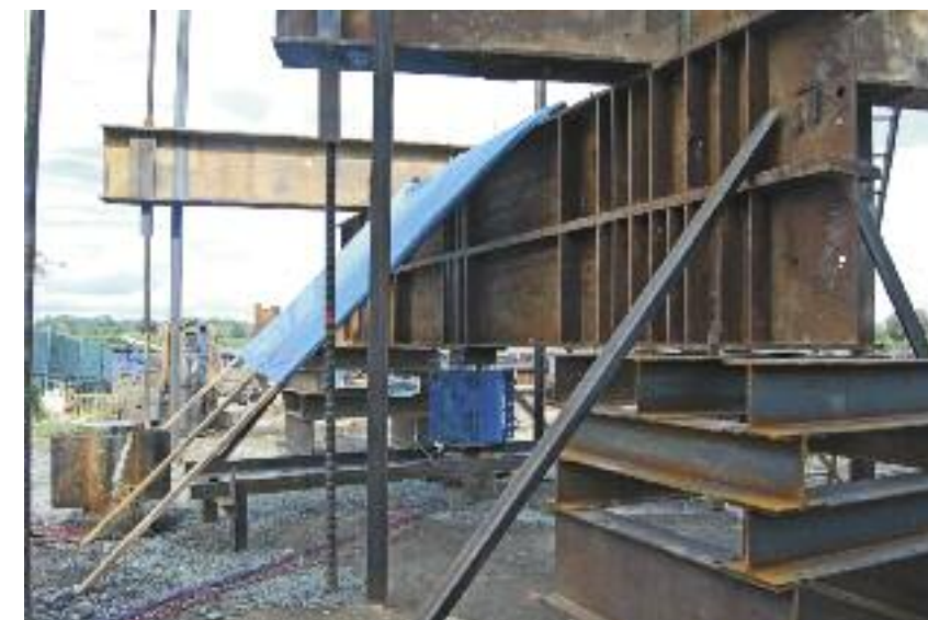
Load test setup.
