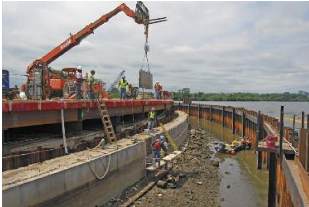
Removal of historic Ashlar facing from Seawall.
