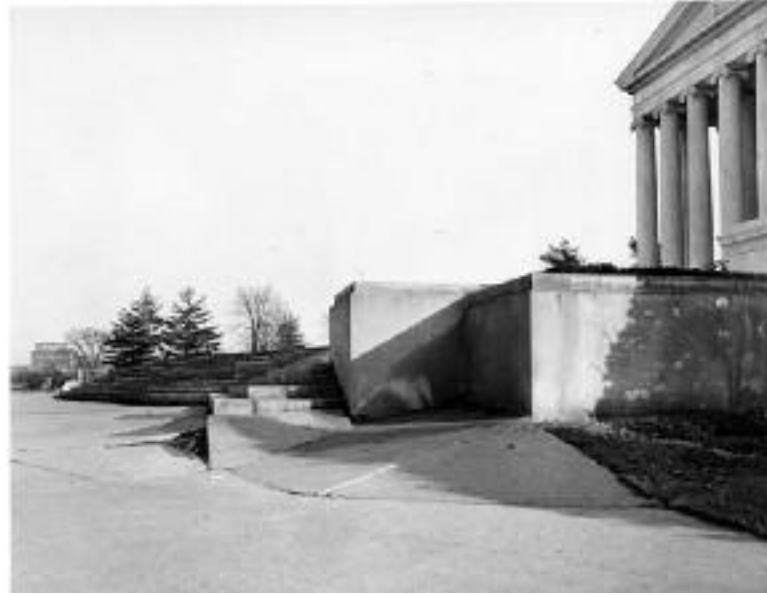
West end of Memorial Stairs. By the 1950s, the North Plaza on grade had experienced significant settlement (the Memorial steps are supported on piles). Source: National Park Service Archives.
