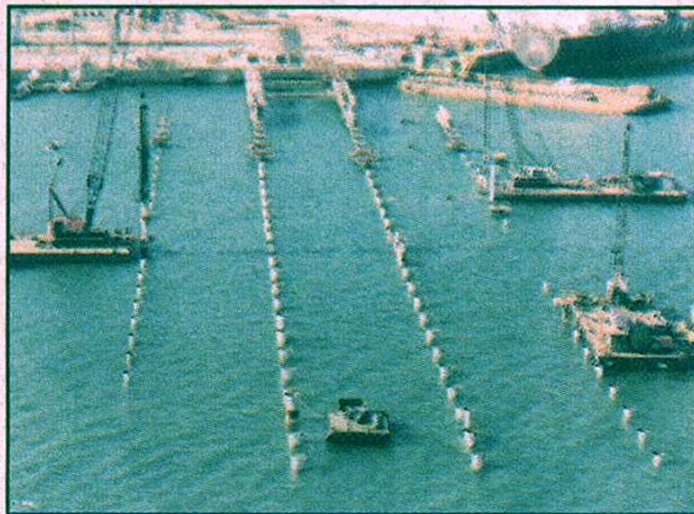
Construction work at Richards Bay jetty
