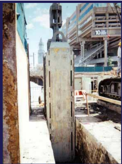
Excavating Immediately Adjacent to a Several Story Building
