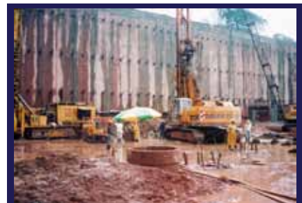
Exposed Wall Constructed under KB Slurry
