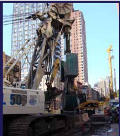
Excavating on 2nd Avenue Subway Expansion in New York City
