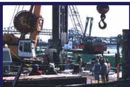
Excavating Panels on a Barge at Harbor Front
