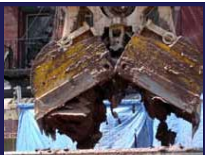
SlurrySMART Stabilizing a Fluidizable Silt in NYC
