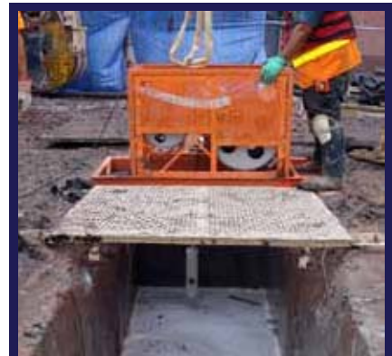
Koden being Dropped into Panel Immediately after withdrawal of Grab
